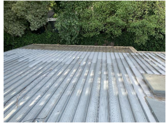
The repaired roof and rust protection completed.
