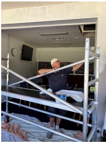
The new mobile scaffold/work platform getting a workout.
